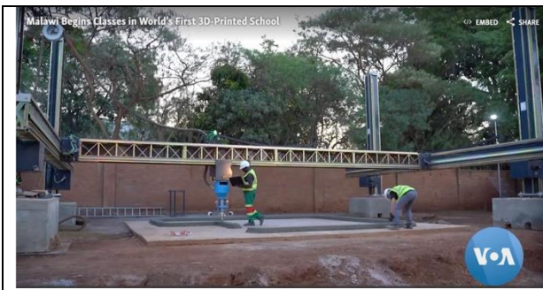
Figure B6.1: 3d printed classrooms in Malawi (2021)
